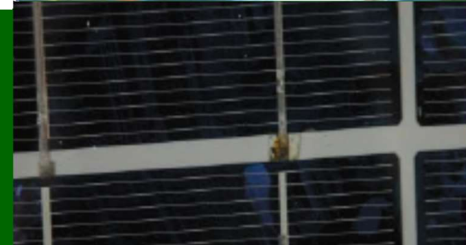
Corrosion inside laminate in salt spray!
